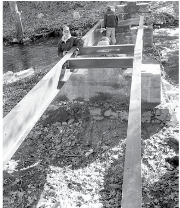
Volunteers place beams for Eightmile River footbridge, late December 2015
