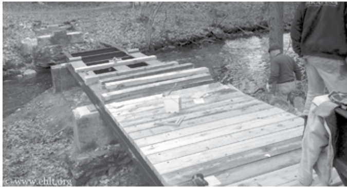
The first decking secured into place, late December 2015
